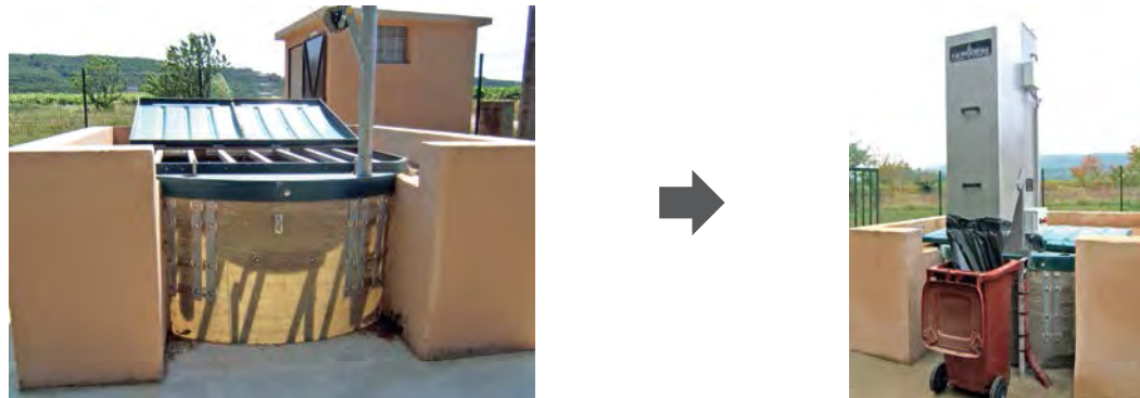
✓ Installation of a Bar Screen Type SG400 on a polyester station
