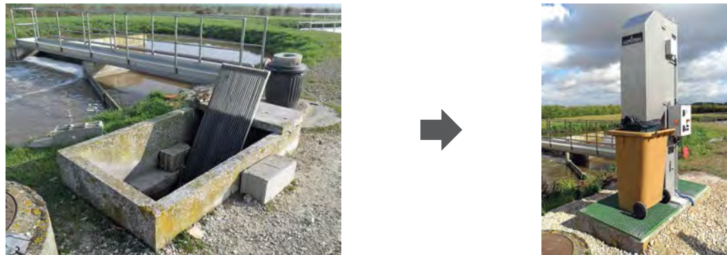
✓ Replacement of a manual screen by a Bar Screen Type SG400
